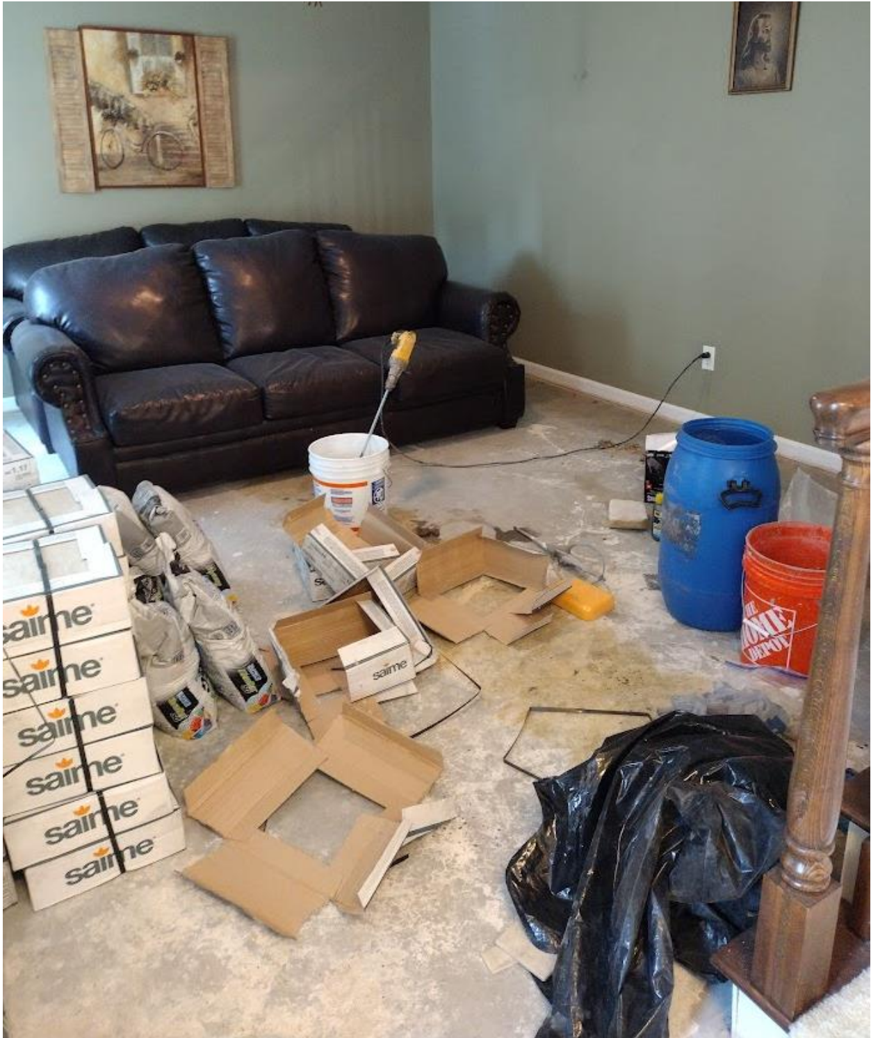
Thinset on brick porch, Photo 1.
