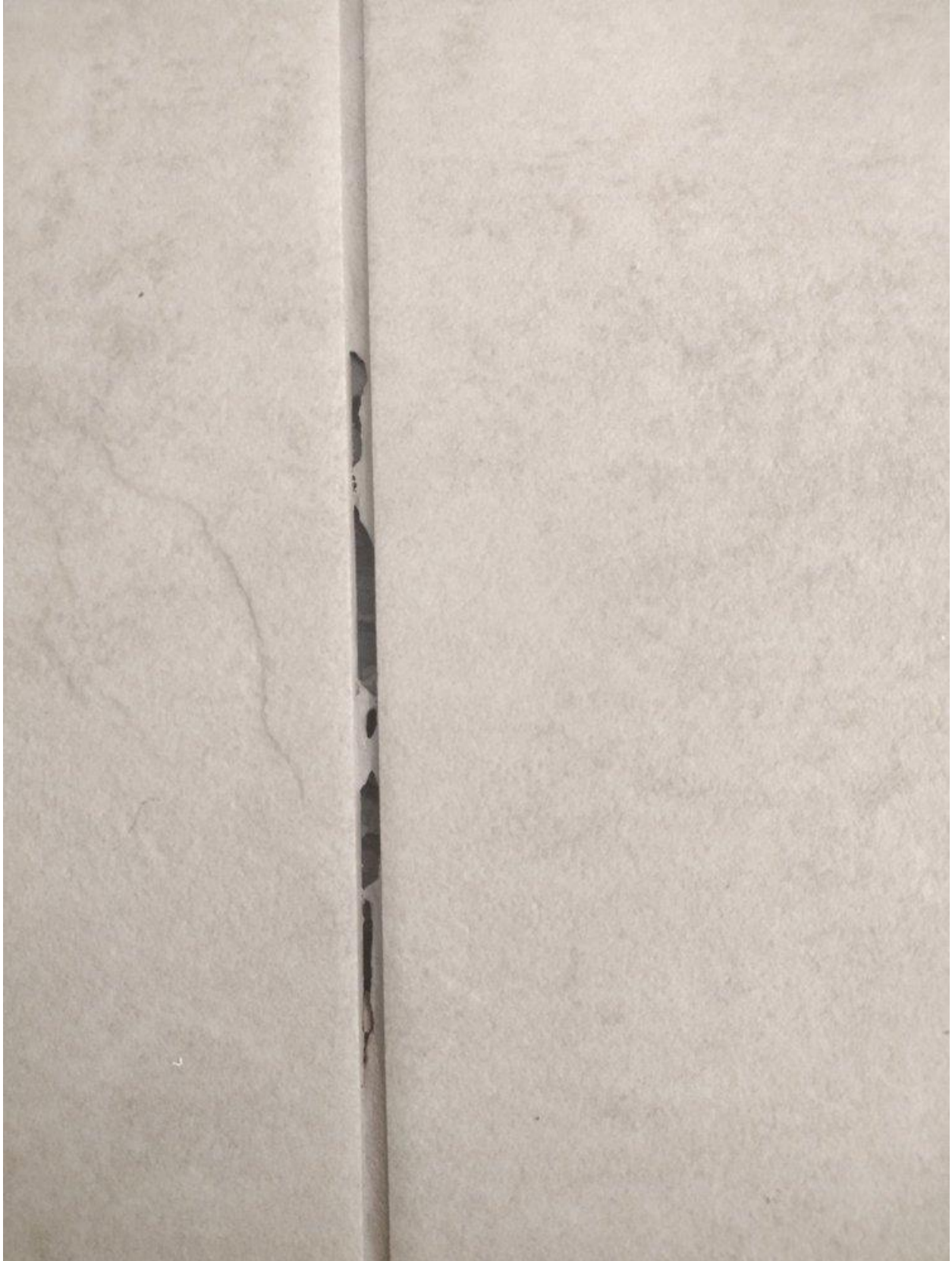
Grout holes, Photo 3.
