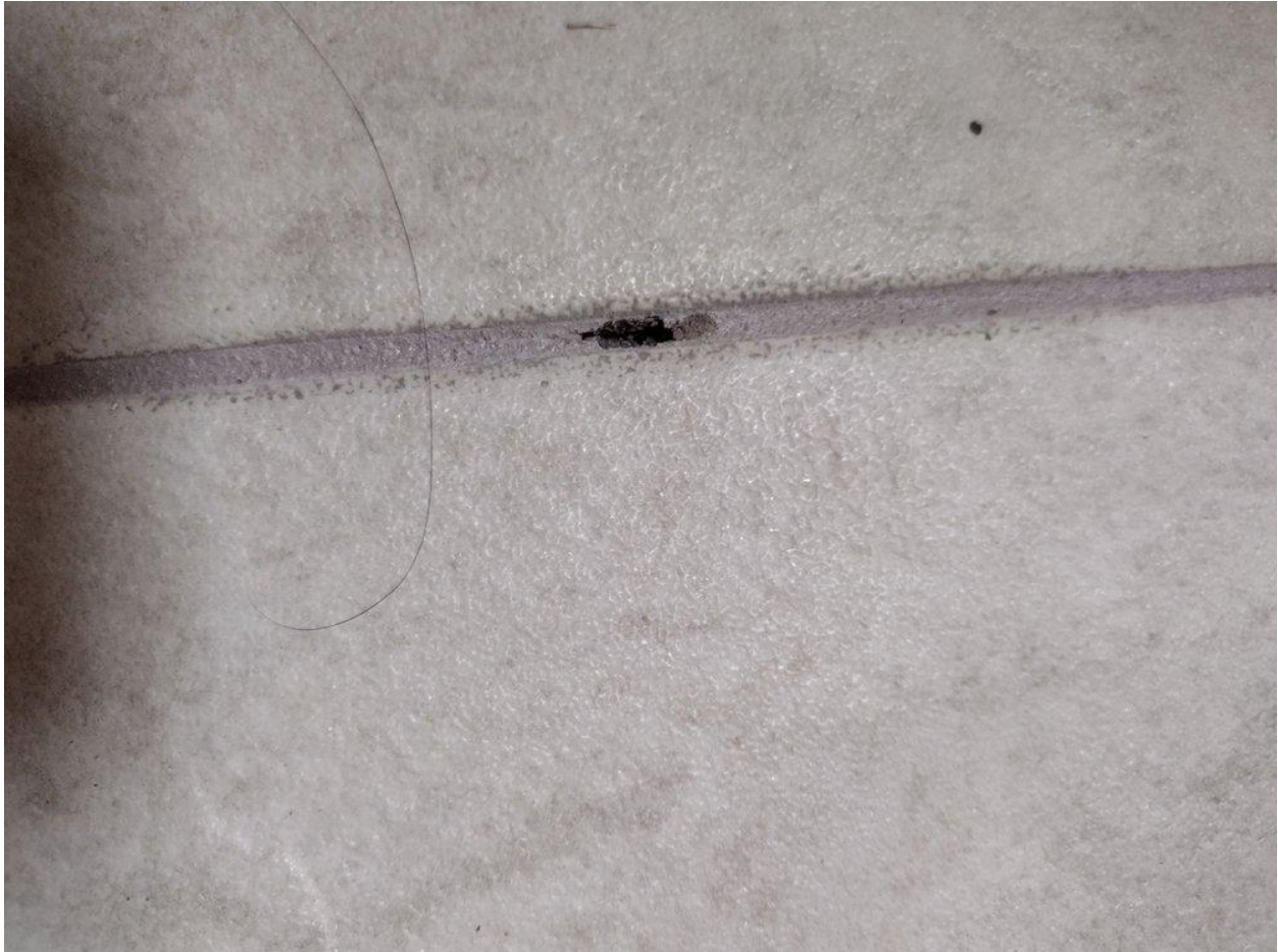
Grout holes, Photo 1.
