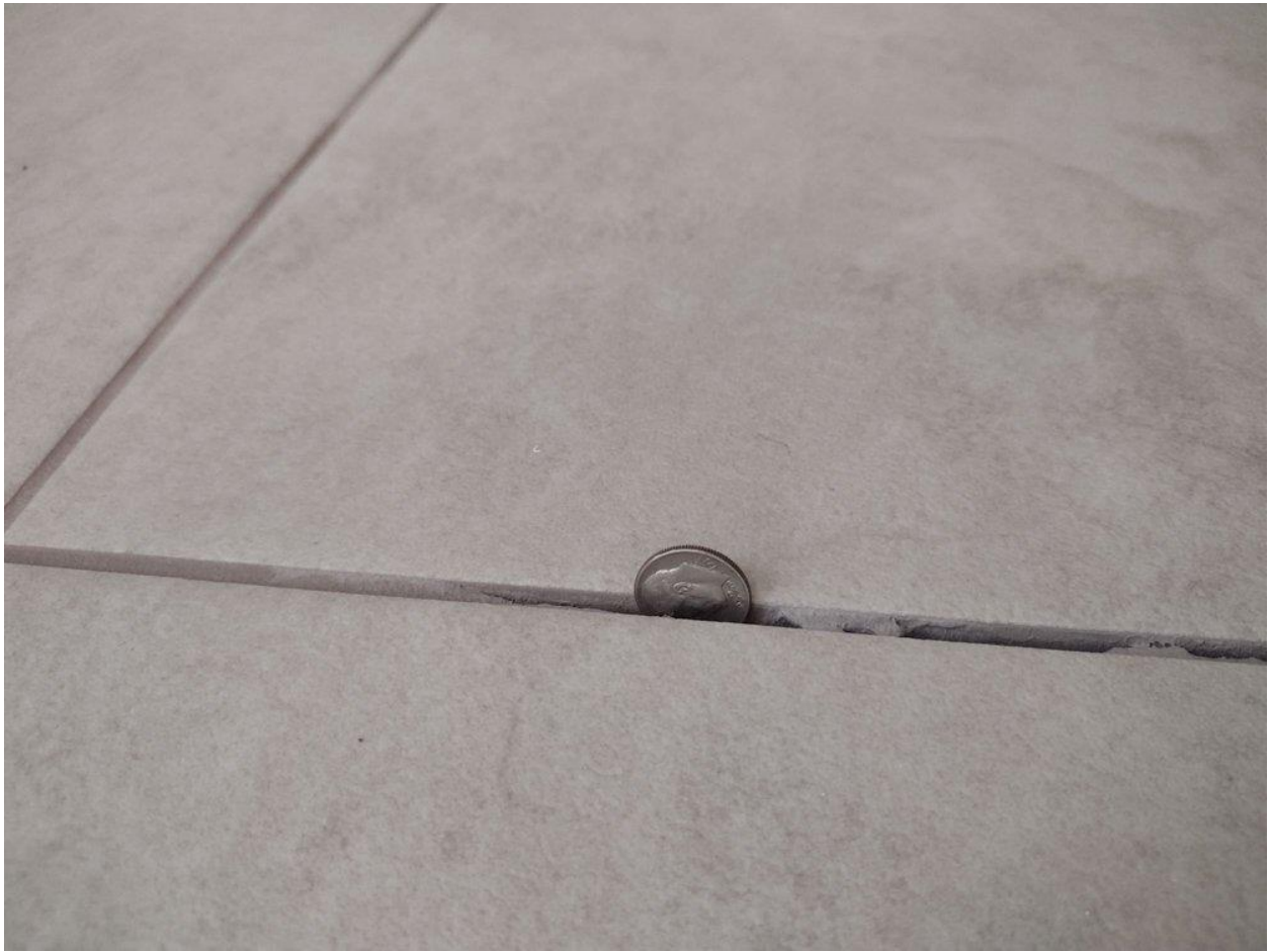
Grout holes, Photo 4.
