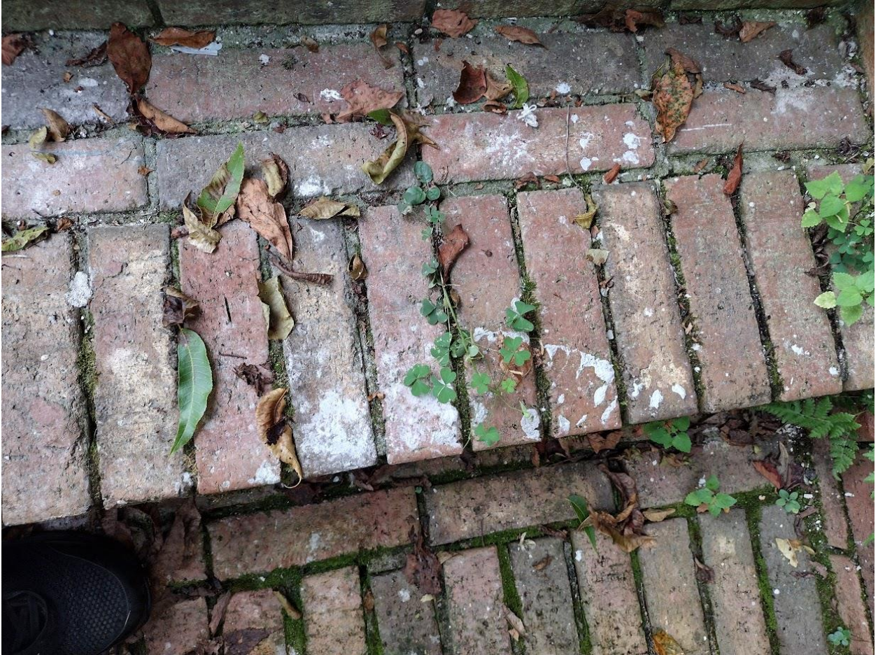
Thinset on brick porch, Photo 9.
