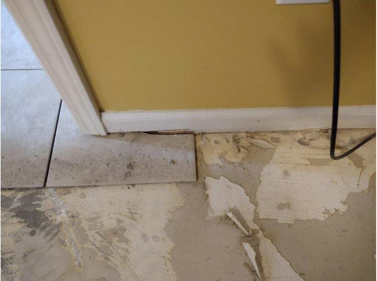
Tile installed over paper, Photo 1.
