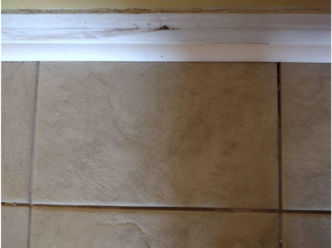
Grout holes, Photo 5.
