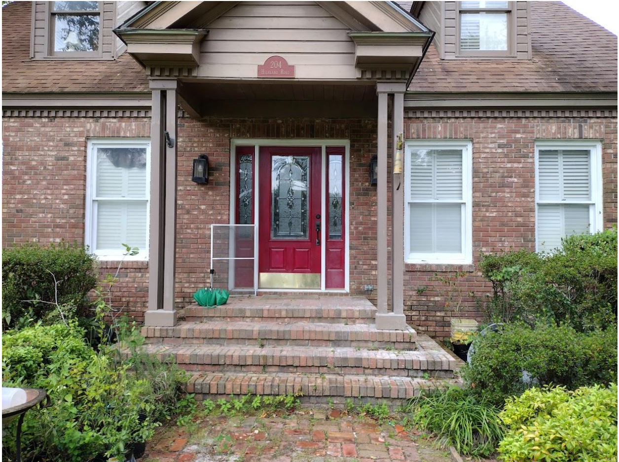
Thinset on brick porch, Photo 4.
