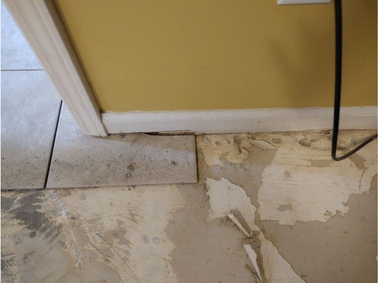
Tile installed over paper, Photo 1.
