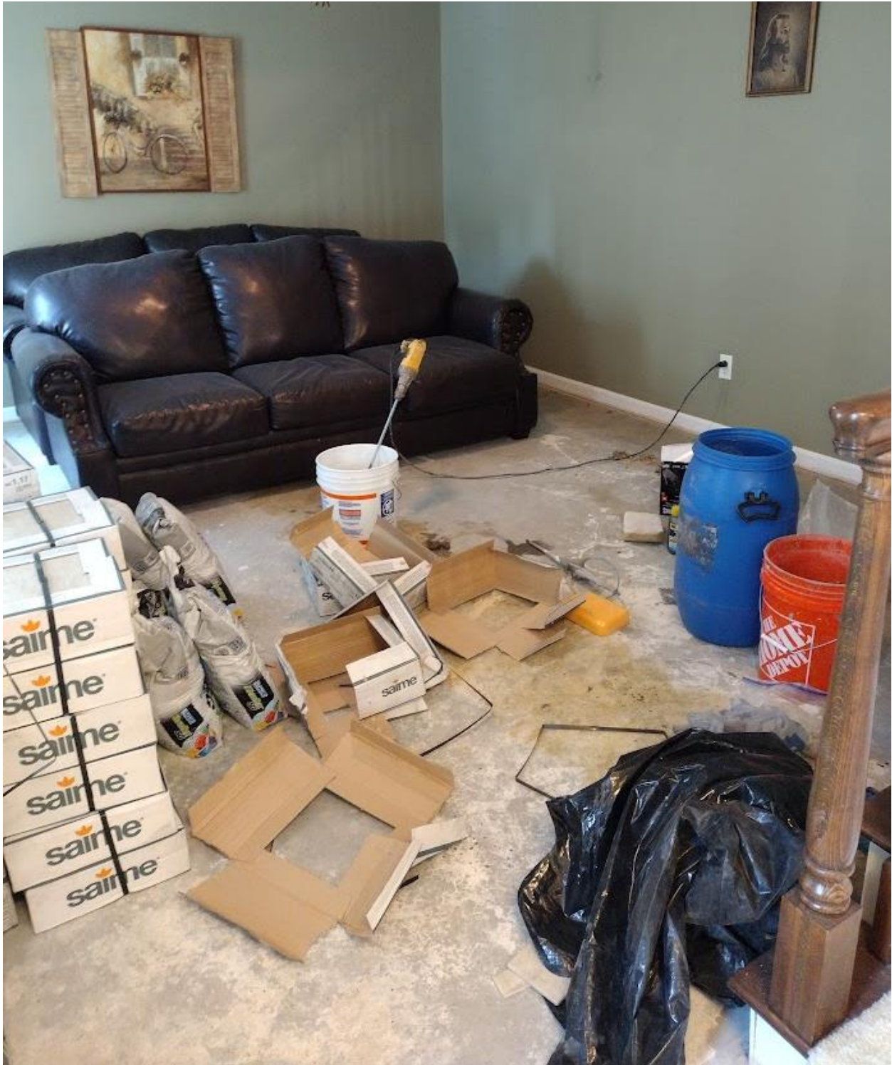
Thinset on brick porch, Photo 1.
